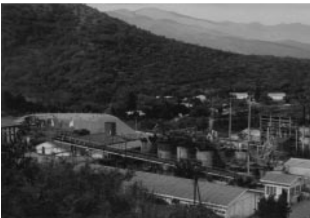
Figure 3 A photograph of the first production-scale biooxidation plant for the treatment of gold-bearing arsenopyrite ore. The plant was commissioned at the Fairview mine, Barberton, South Africa and was originally designed to treat 30% of the mine's production. In 1991 this demonstration plant was extended to treat the full production of approximately 40 tons of concentrate per day. (By kind permission of Gencor Ltd, Johannesburg, South Africa.)
